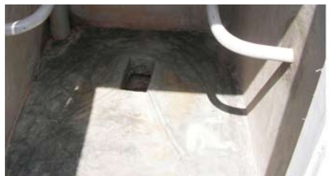
The newly constructed accessible pit latrine at Kiboga Progressive Senior Secondary School
