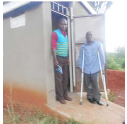
A ramp at the entrance of a PWDs latrine at Kapeke Seed School
