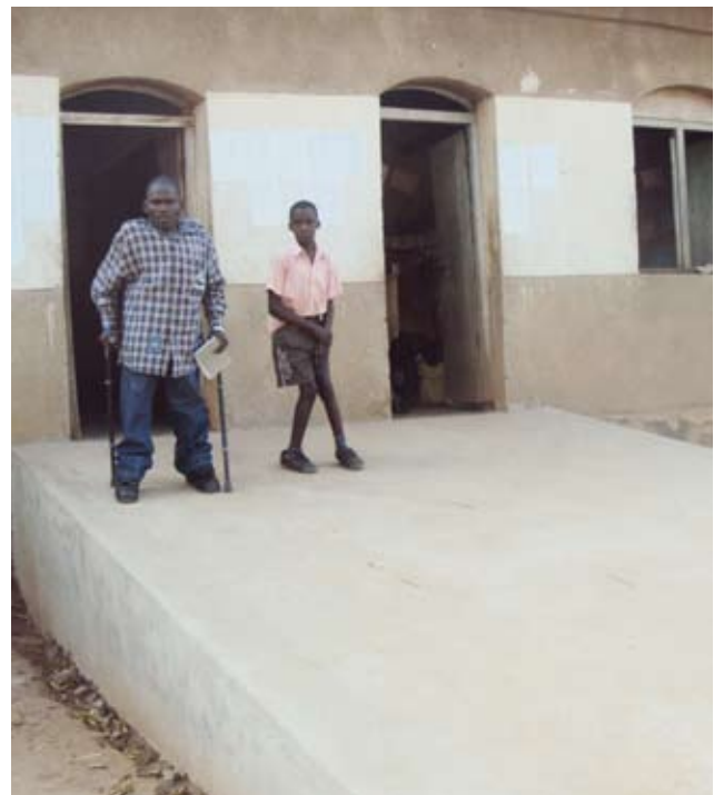
Mukasa and Amanyā at the newly constructed ramp leading to his class
