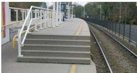
Graphic 2: One platform with two heights (Amsterdam and Utrecht, both metro/light rail vehicles)
